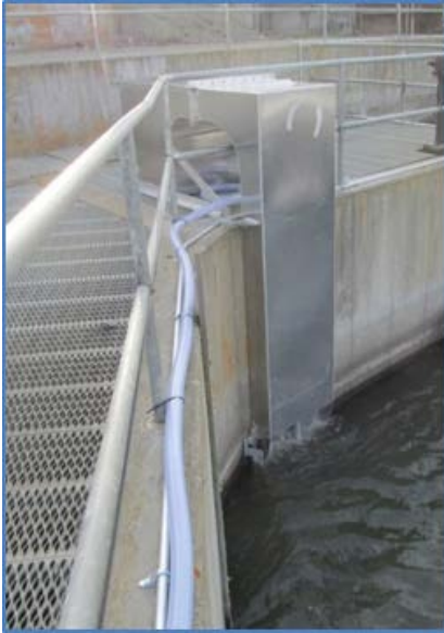
Photo 1. Vertical Wetted Wall Lamprey Passage Structures installed at Prosser Dam (left - Lower Structure, right - Upper Structure). The vertical center guide pipe allows lamprey that are passing along the ladder wall from either directions to sense the flowing water.
