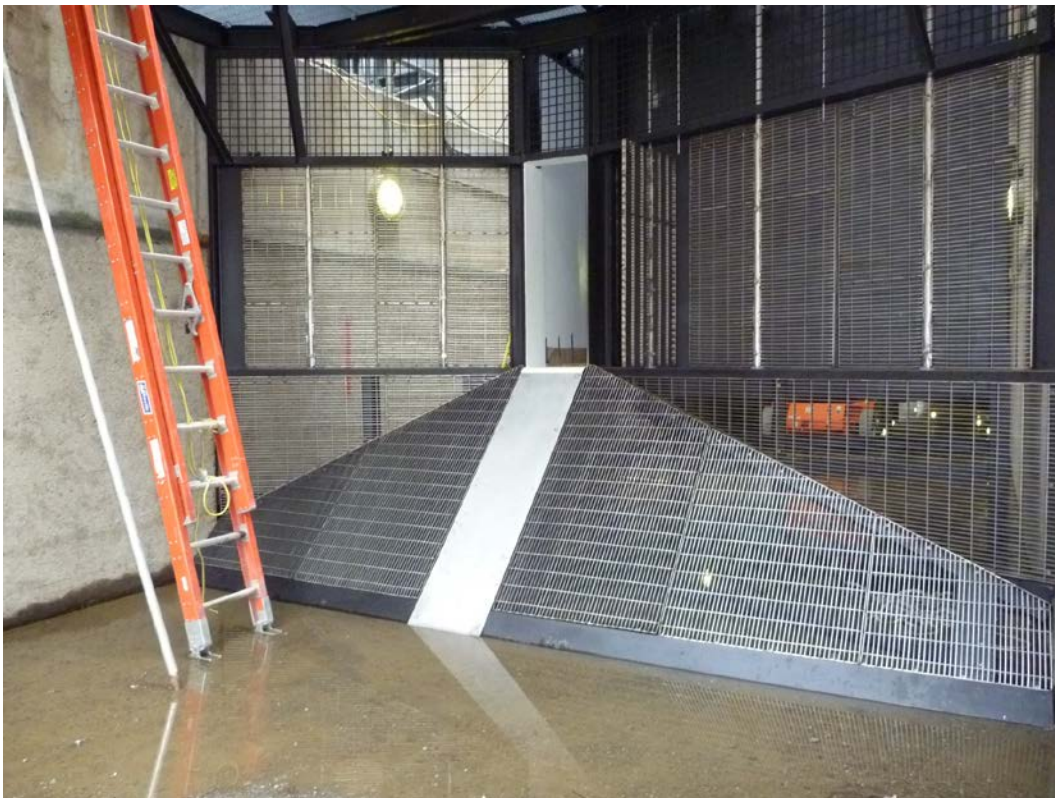
Figure 3. Priest Rapids fishway- approach to counting window and modifications for lamprey.
