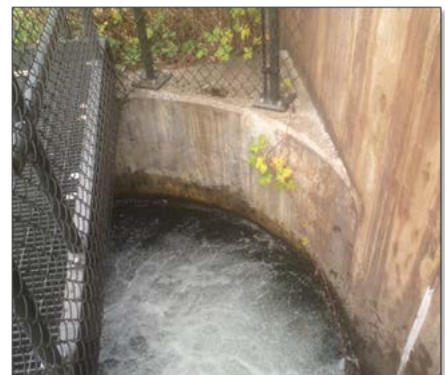
Figure 1. Photos of Pacific Lamprey passage design elements of the River Mill fish ladder. Rounded entrance and filled entrance gate bulkhead slot (left), chamfered orifice and weir (middle) and rounded ladder corner (right).
